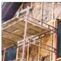
Roof and Wall Insulation
